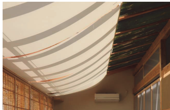
Figure 10 Roll blinds under skylights.
