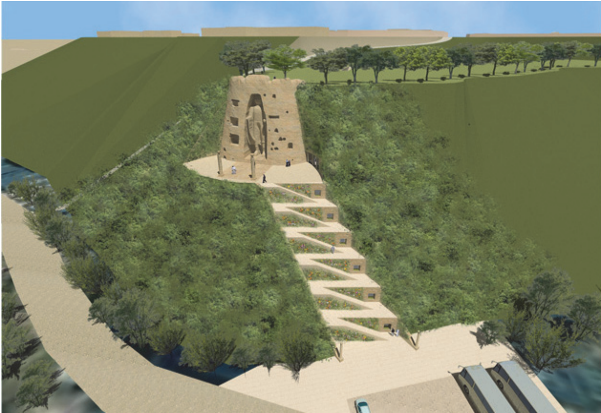
Bird's-eye view of the proposed monument from the north direction: A one-third scale of the Eastern Buddha is constructed on the platform halfway up the hillside. The outdoor steps connect the foot of the plateau and the platform.
