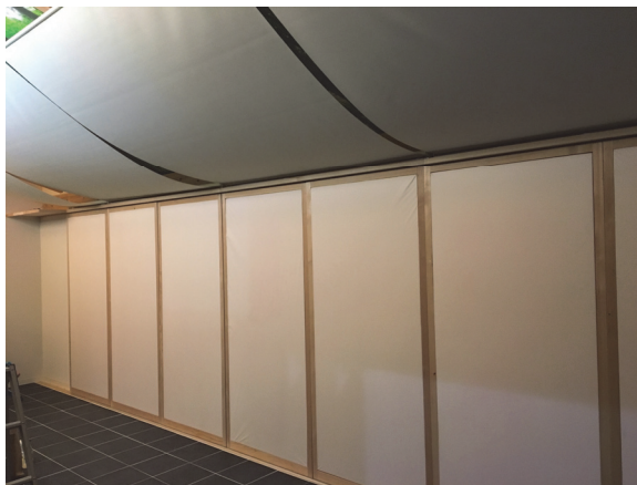
Figure 7 Window shades installed inside windows for insulation.
